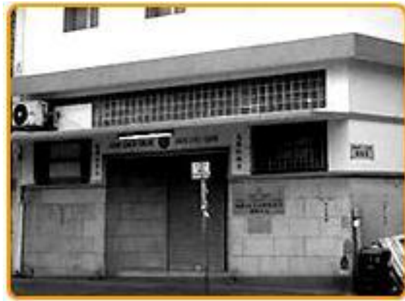
The No.9 Arran Street single-storey premises erected by Kowloon Rotary Club in 1951
