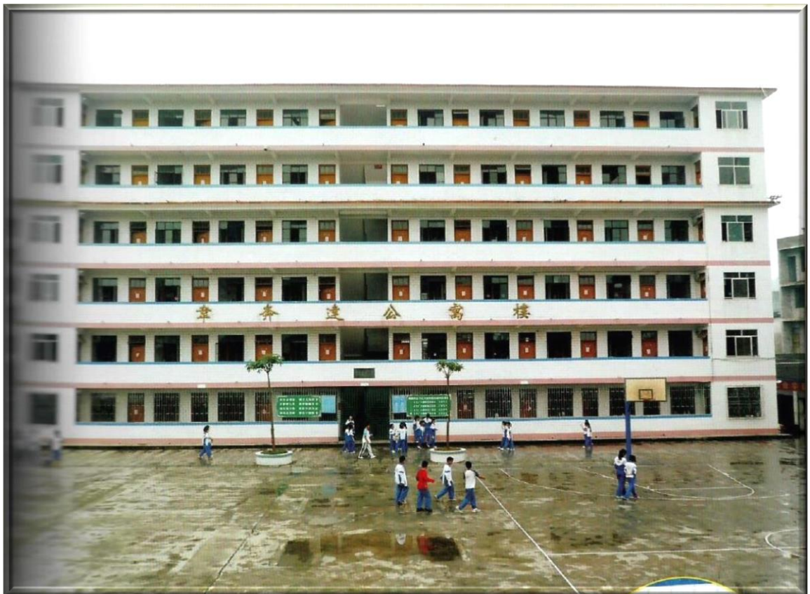
2005 – Bill Benter donated the construction cost of the [Benter House 韋奔達公寓樓] Student Dormitory of Du'an Yao Ethnic Experimental Middle School
