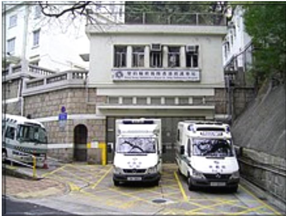
St. John Ambulance depot at 2 Tai Hang Road, Causeway Bay, Hong Kong Island.
