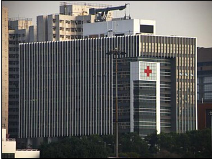
Hong Kong Red Cross Headquarters Run Run Shaw Building 香港紅十字會總部邵逸夫樓
