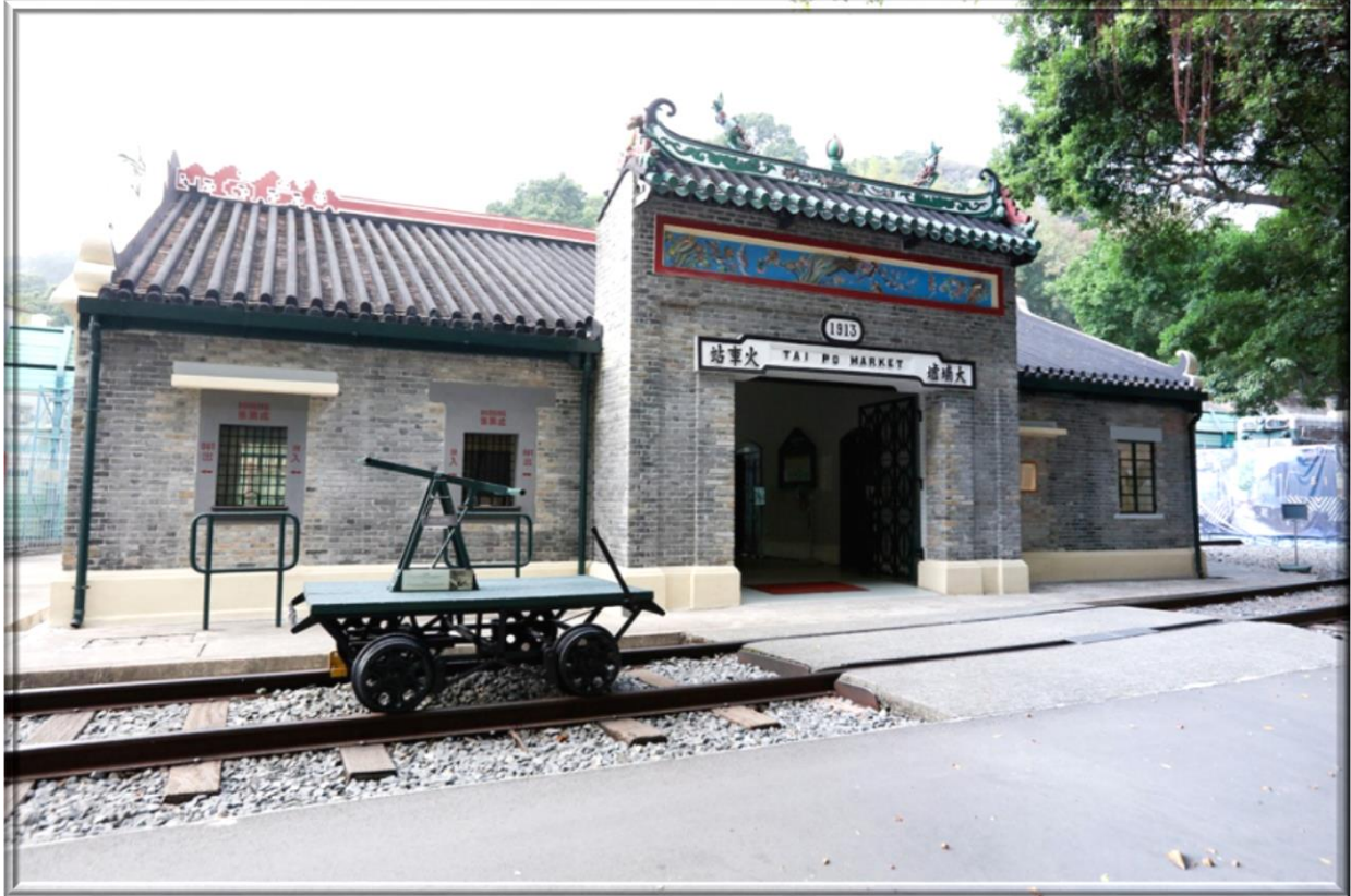
Former Tai Po Market Railway Station -- in its classical Chinese architecture built in 1913
