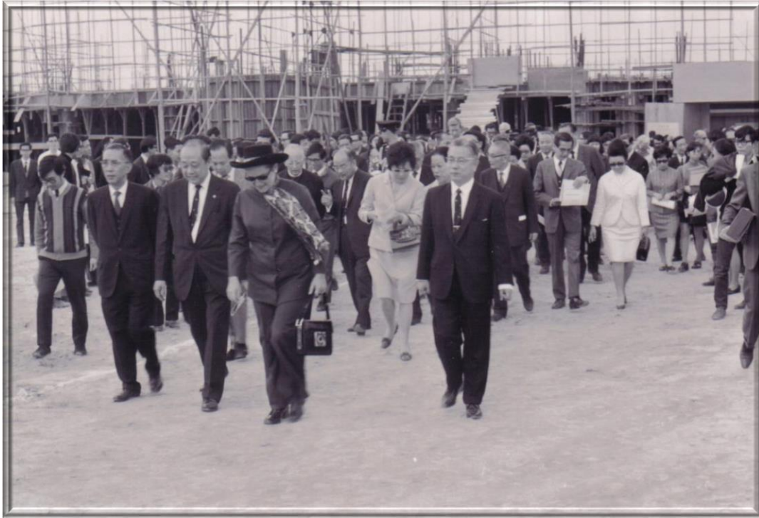
1971年3月—香港聯合書院董事會主席馮秉芬議員(左二)視察位於香港中文大學沙田校園內的書院新校舍建築工地。 March 1971 – The Honourable Kenneth Fung Ping-Fan (left 2), Chairman of the Board of Trustees of the United College, inspects the new construction site of the College located inside The Chinese University of Hong Kong campus in Shatin.
