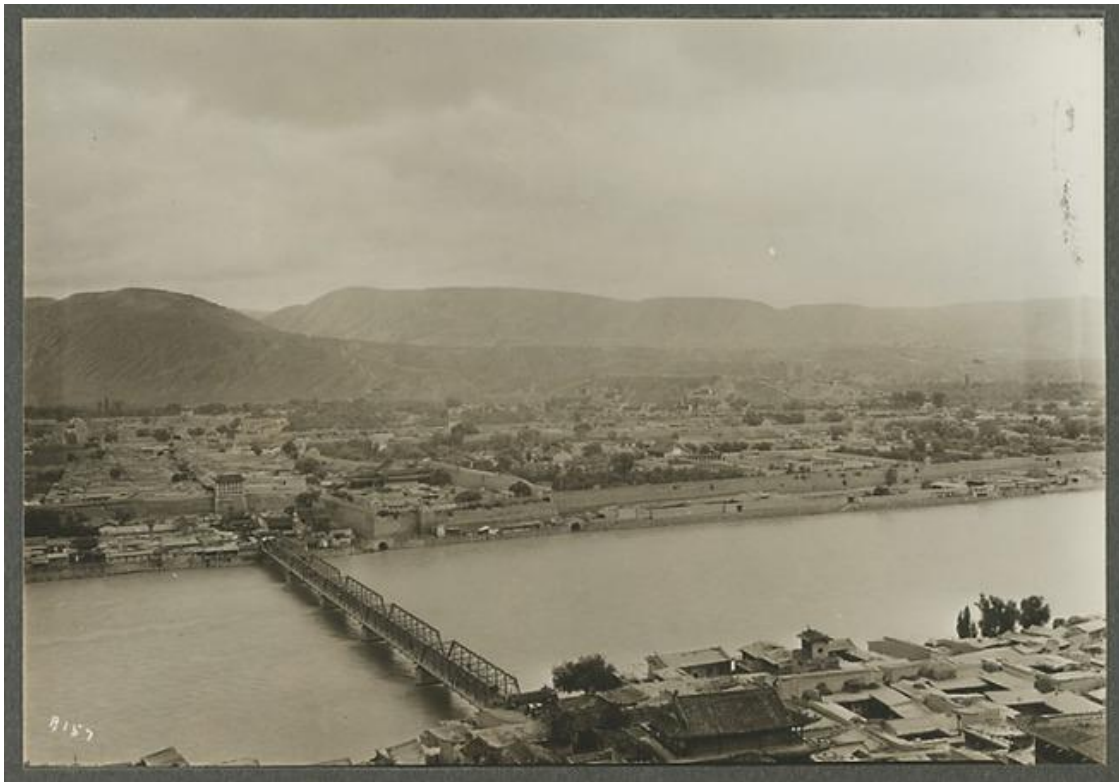
The American bridge over the Yellow River, Lanchow
