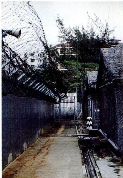
Ominous chain link fences and barbed wire surround the closed camps.
