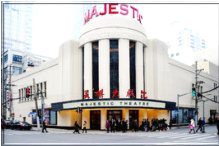
1941 年建成的美琪大戲院 (與范文照聯合設計) -- 上海市靜安區江寧路/奉賢路, 上海市優秀近代建築保護單位 Majestic Theater (1941) (Joint-design with Robert Fan) -- Intersection of Jiangning Road and Fengxian Road, Jingan District, is now an excellent modern architecture protection unit in Shanghai
