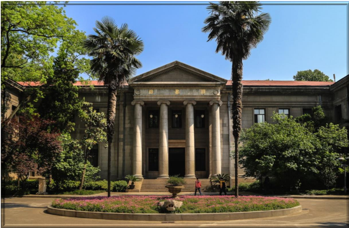
允元實業公司的 1923 年作品 --- (南京) 國立東南大學孟芳圖書館 A remarkable project by Lam Glines & Company in 1923 --- The Meng Fang Library Building of the National Southeast University located in Nanking (Nanjing)
