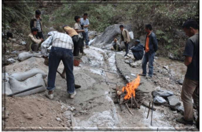
Villagers working on channel at the water source to collect water in the sediment tanks before entering the pipes.
