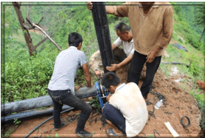
Villagers connecting the water pipes.
