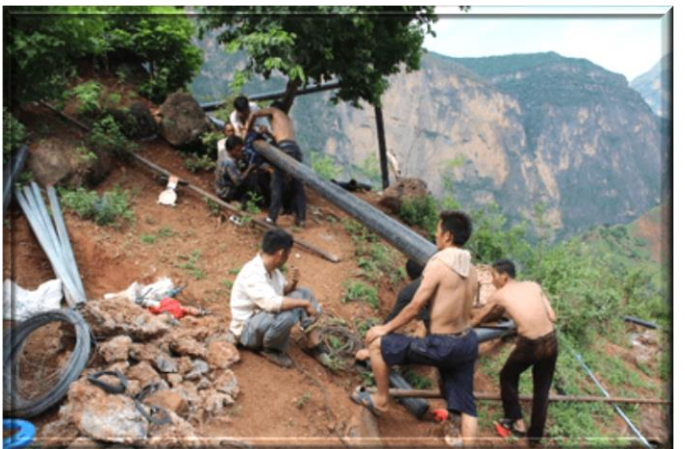
Villagers connecting the water pipes.
