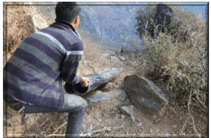
Villagers had to carry 160mm PE Pipes with the length of 4M manually up to the water source.
