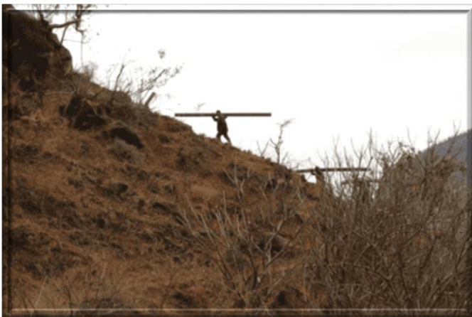
Villagers had to carry 160mm PE Pipes with the length of 4M manually up to the water source.
