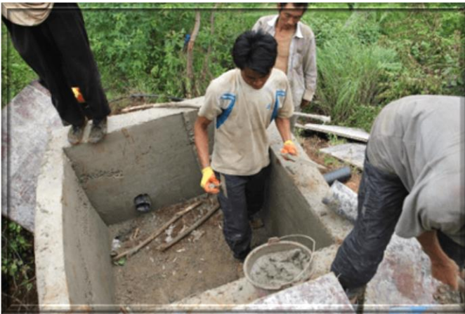
Building of the sedimentation tank
