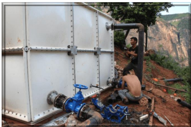
Connecting pipes from water tanks to every household.
