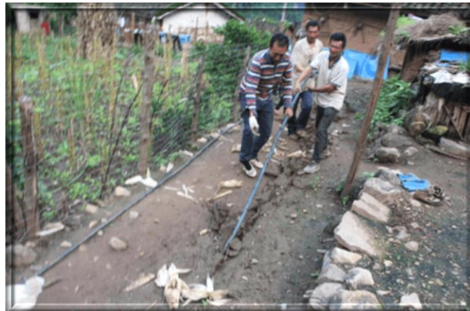
Connecting pipes from water tanks to every household.
