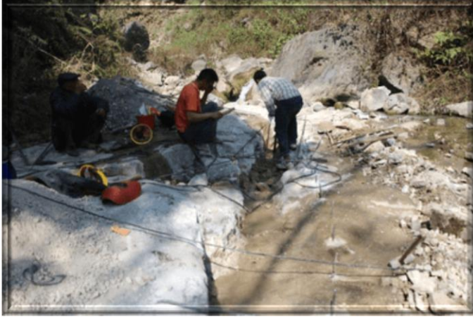
Villagers working on channel at the water source to collect water in the sediment tanks before entering the pipes.
