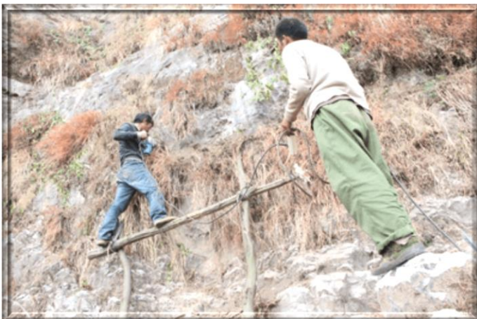
Connecting the pipes and fixing the pipes onto the wall of the cliff.
