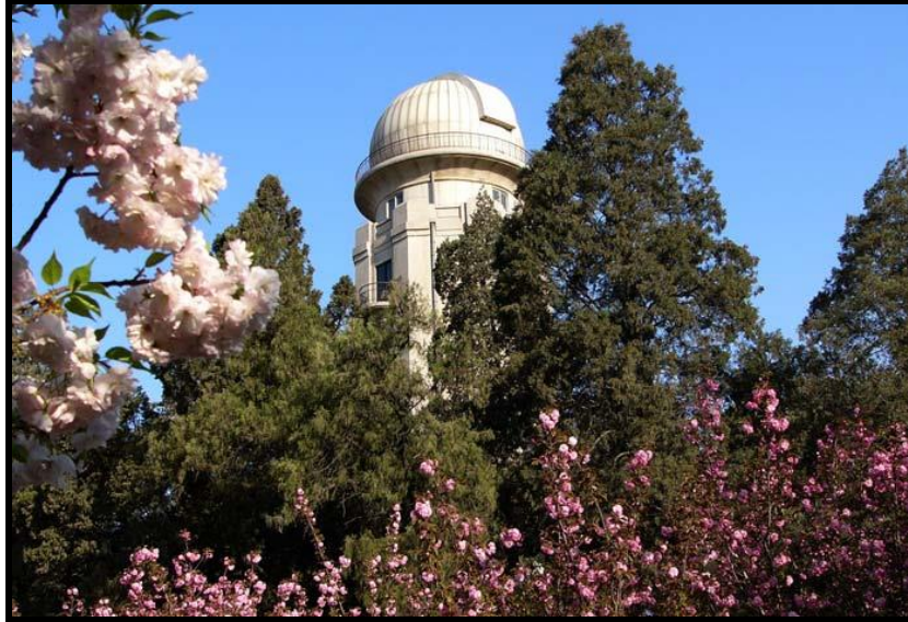
1931 年建成的國立清華大學氣象臺 Observatory of National Tsinghua University built in 1931
