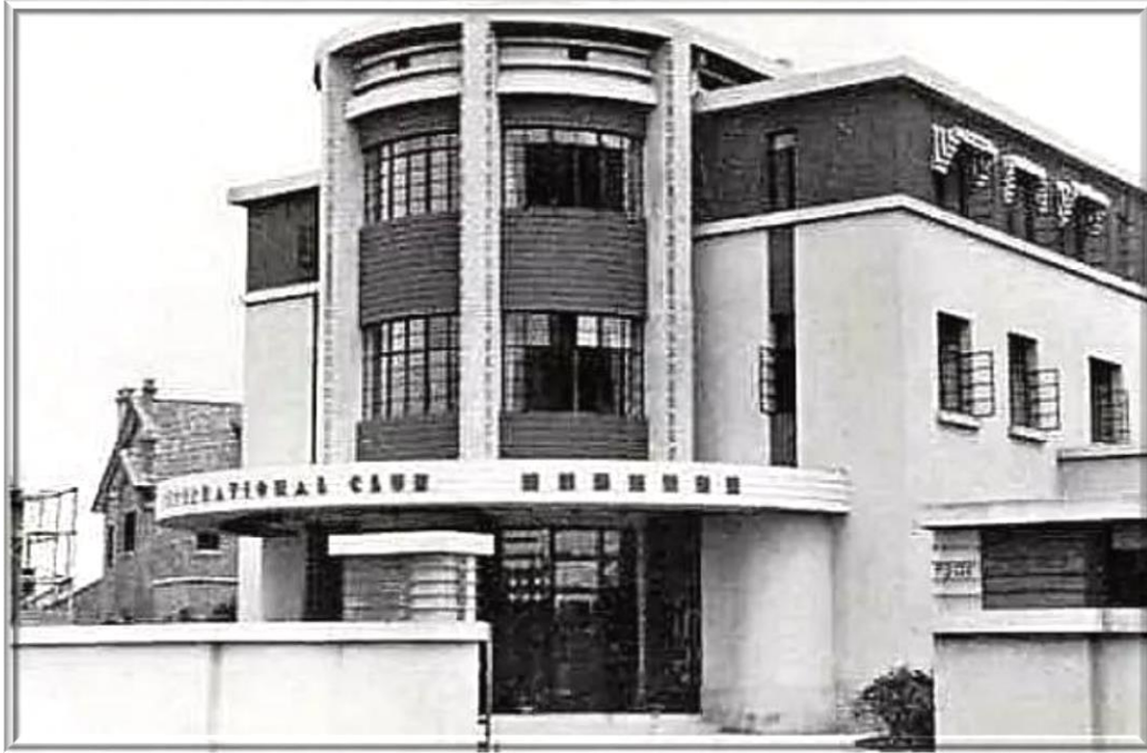
The regular weekly meetings of the Nanking Rotary Club was held in this International Club (國際聯歡社), in the nation's capital Nanking, which was the clubhouse of the Foreign Affairs Ministry. The complex was completed in 1936 by the architecture firm of Tientsin Rotarian Kwan Sung-Sing (天津扶輪社社員關頌聲).
